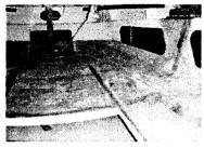
Fig 2 Boat upside down and inside glass stripped ready for new stiffeners.
